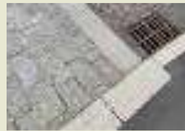
Granite setts in contrasting colour (example uses include drainage areas in verges and at junctions)
