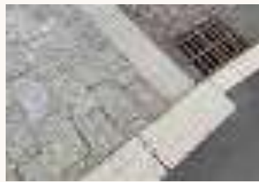
Granite Setts in contrasting colour (example uses include drainage areas in verges and at and junctions)
