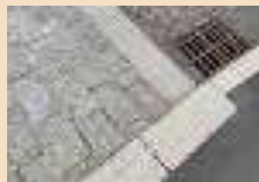
Granite sets in contrasting colour (example uses include drainage areas in verges and at and junctions)
